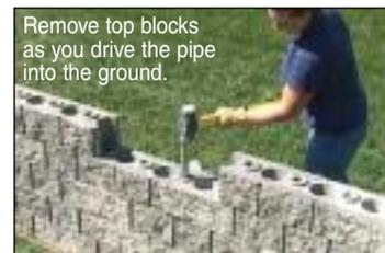
Remove top blocks as you drive the pipe into the ground.
