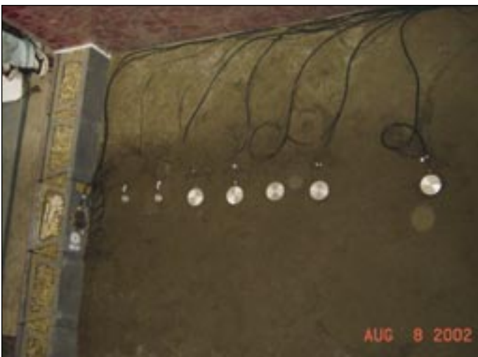
Load Transducers for Measuring Vertical Earth Pressure
