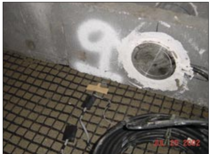
Earth Pressure Transducer Behind the Block and Strain Gages on the Geogrid
