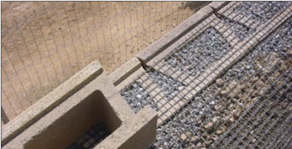
Allan Block reinforced with Huesker geogrid.
