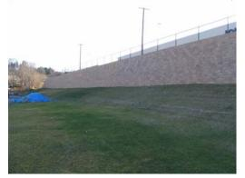
A typical design section for a wall such as this one would be similar to this section from AB Walls 2007. The standard grid lengths would be around 60% of the total wall height and the top few layers of grid, depending of the wall height, would be lengthened to 90% of the total wall height due to the paved surfaces above. It is common practice to lengthen top grids for three distinct conditions:
