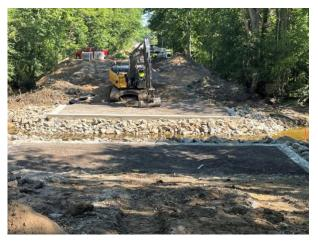
Segmental Retaining Walls (SRW) units have several advantages over a CMU especially with regards to durability and dimensional tolerances which was also a factor. Midland like most of the northern US, experiences harsh winters and the county needed a product that would last over the long term.
