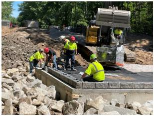
OHM Advisers eventually settled on the <u>AB Vertical</u> that would keep the structure's footprint closely in line with the existing road further reducing the amount of excavation for the project.
