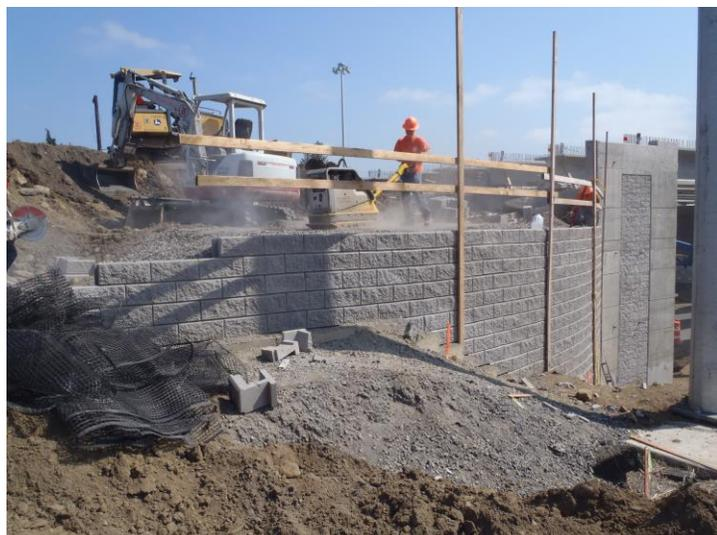
monitor and control the wall alignment during construction. Careful layout and close attention to proper leveling techniques ensured that the walls properly aligned with the bridge abutments when all was said and done.
