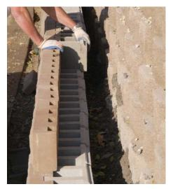
When facing the old SRW wall with AB Fieldstone and no-fines concrete, Harris and his crew were off to the races since they could stack the units and place the No-Fines as fast as they could. The placement of No-Fines concrete requires only minimal rodding to consolidate and can be poured in 2-course lifts. The set time is very short which allows work to continue at a high pace. The two-piece AB Fieldstone units are so the workers could place more square footage per day.
