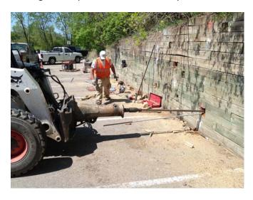
layers in place and then restacked using the new AB Fieldstone units by reconnecting the grid as the wall is reconstructed. This is a complicated process for the installers and takes great care to not damage the
