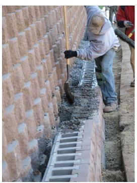
common way by placing grid between the lower courses and bringing it up around the back of the pipe and back to the wall between the next two courses above.
