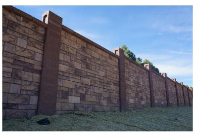
Due to the lack of space for storage and the two major highways that ran parallel with the fence, pallets of block had to be brought to the site daily to keep the project moving forward. To save time on the project, the bond beams were constructed by precasting them off site which allowed a high quality production of the structural bond beams. Since the crew that constructed the bond beams were only focused on the pre-casting operation, the
