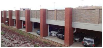
The West practice field would be constructed on grade and the East practice field would be elevated 14 feet (4.3 m) above the surrounding street level. A fence system was needed at the edges of the practice fields for privacy, security, and safety. For the University of Arkansas fence, Polk Stanley Wilcox Architects also needed to incorporate the design of the garage structure with the design of a fence above so the look of the facility would
