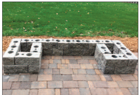
Completed 2nd Course
