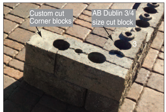
Build Back Wall
