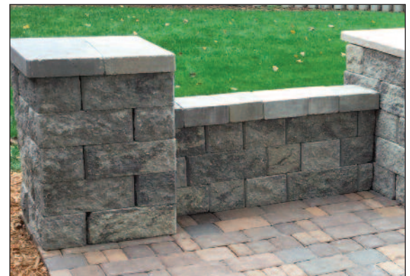
Install Wall and Post Caps
