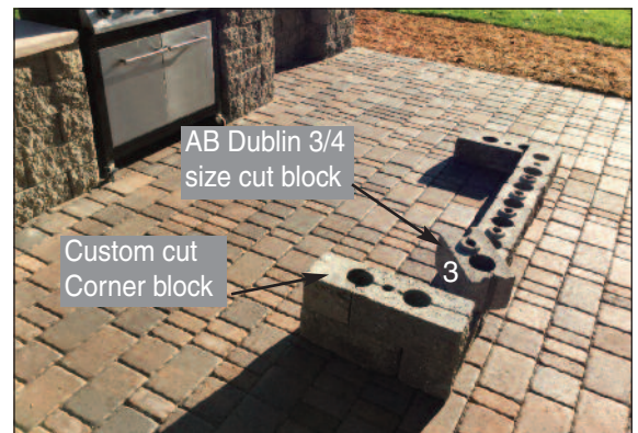
Build Back Wall
