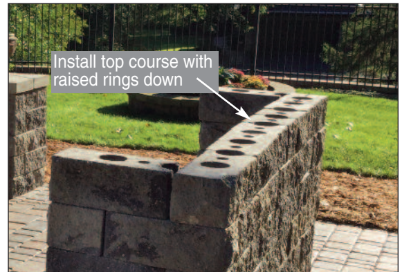
Install Top Course
