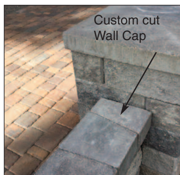
Capping straight walls
