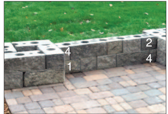
Install 2nd Course of Wall Panel
