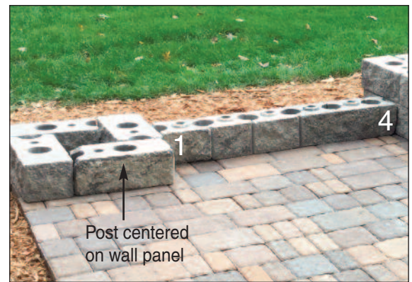
Install 1st course Wall Panel and Post
