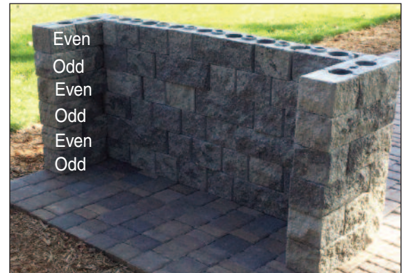
Install Additional Courses
