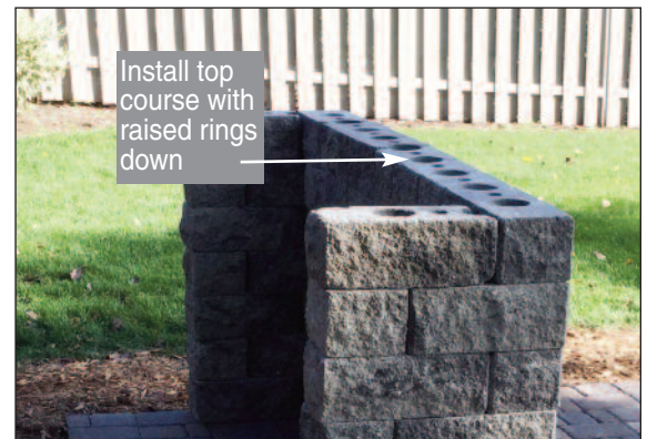
Install Top Course
