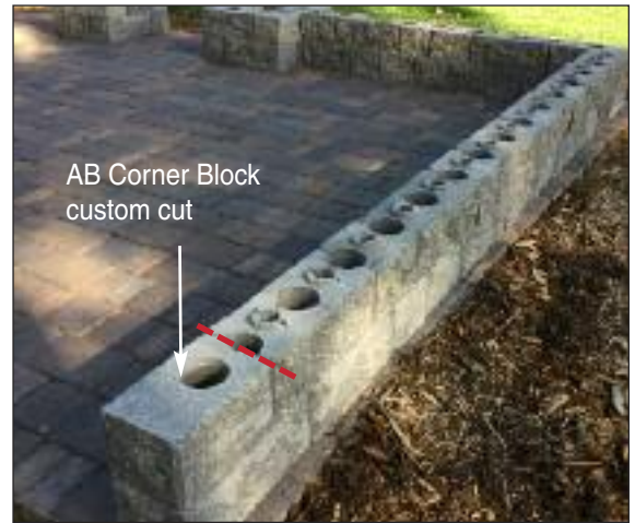
Finishing Second Course
