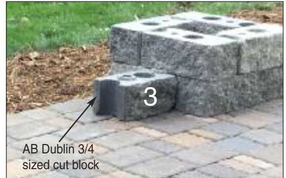
1st block of panel
