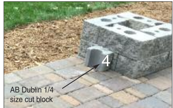
1st block of panel
