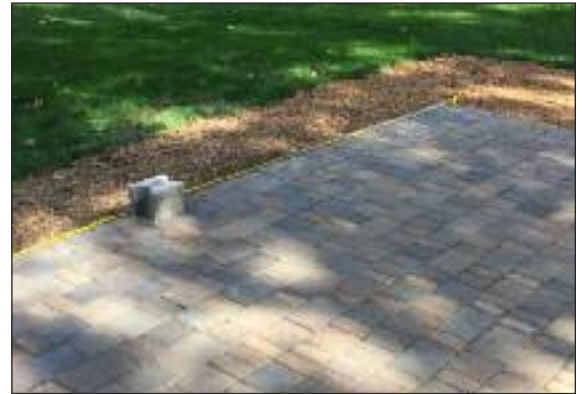
Determine Layout / Install 1st Block
