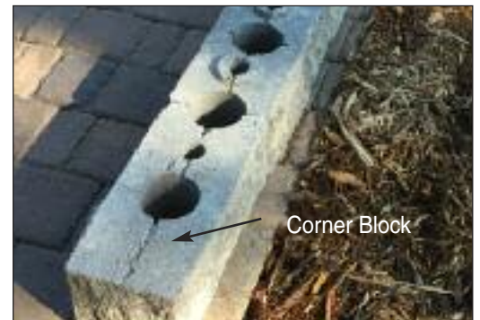
Finish with a Corner Block
