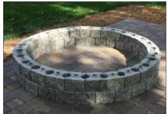
Install 2nd course
