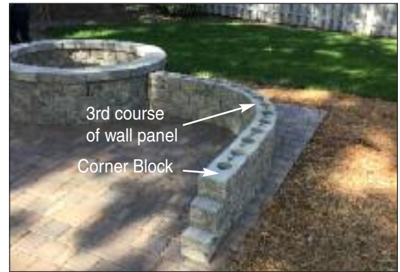
Third Course Wall Panel
