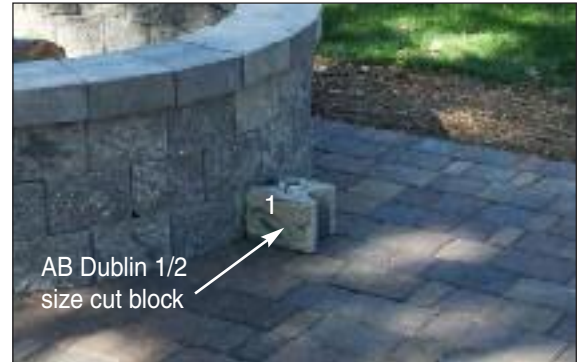
1st block of panel
