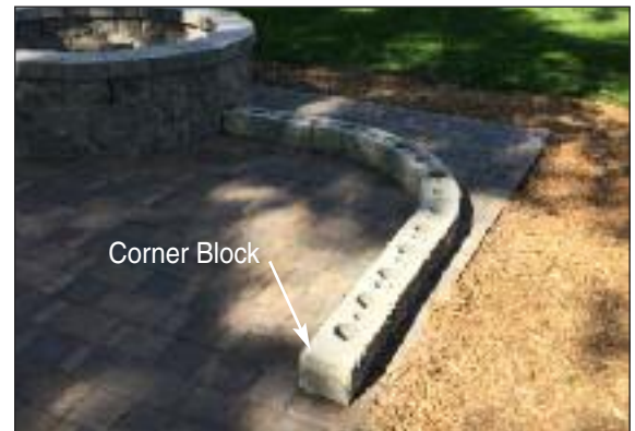
Finish with a Corner Block
