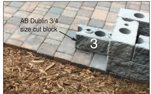
Install cut block to start wall panel
