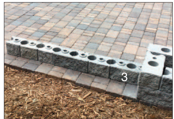
Build wall panel
