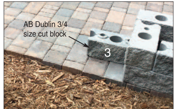
Install cut block to start wall panel
