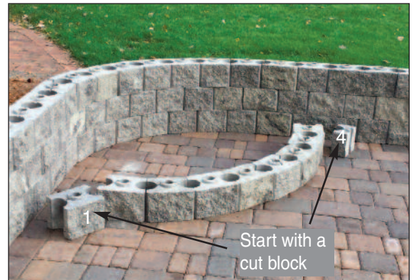
Inside front wall
