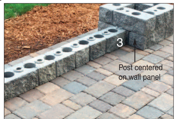
Place a cut block at next post location
