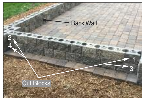
Second Course Wall Panel
