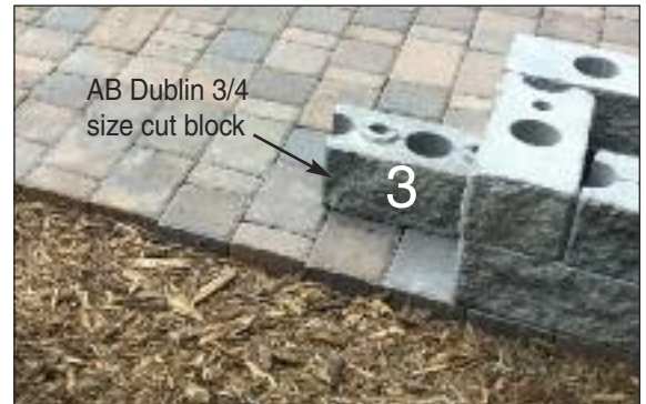
Install cut block to start wall panel
