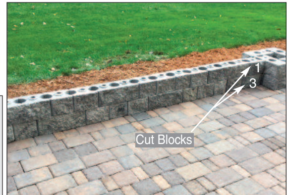
Second Course Wall Panel
