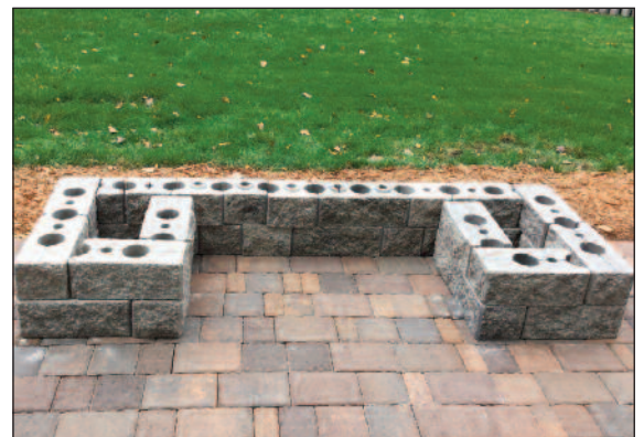
Completed 2nd Course
