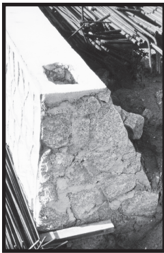
Mortared Stone Gravity Wall Malaysia
