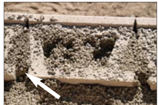
Remove one back wing per block.
