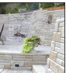
Use a compactible rock or sand behind the entire wall. This provides a fill that is less likely to settle over time. Compact the entire area behind the blocks making a minimum of two passes with a walk behind plate compactor.
