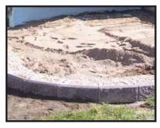
Make minor adjustments by using a dead blow hammer or by placing up to 0.5 in. (13 mm) of course sand under the blocks. Keep in mind irregularities in the base course become larger as
