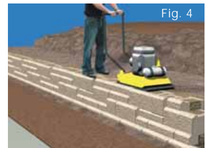
Install the second row of the two course pattern. Backfill and compact, adjust for level as necessary.
