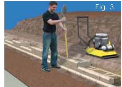
Backfill the blocks and behind the blocks. Use a shovel handle to compact inside the blocks.
