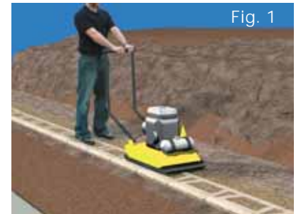
Install, level and compact base course and backfill behind wall.
