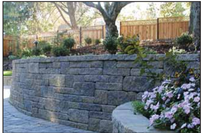
This project uses 2 two course patterns and a one course pattern to complete the wall.
