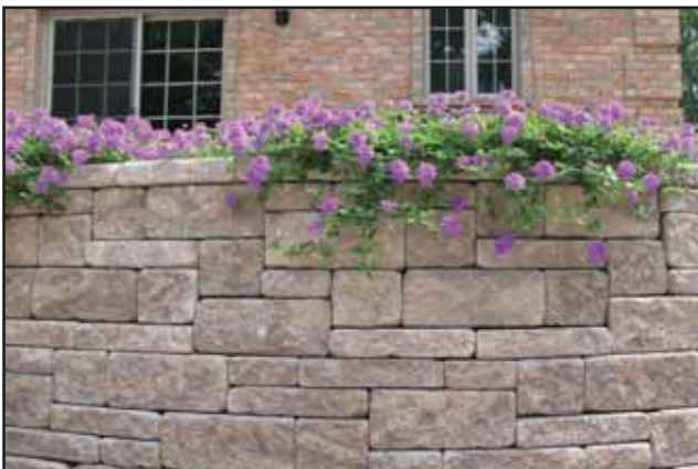
This project uses a two course and a three course to complete the wall.
