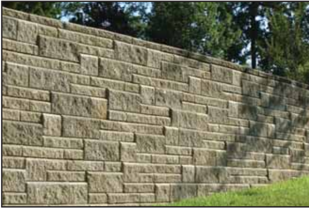
This project uses 4 two course patterns to complete the wall.
