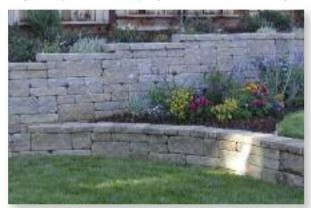
**Outside Curves** are created by removing one or both of the wings on the back of the block to create a smooth and flowing radius.
