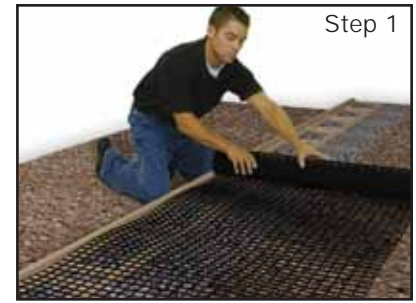
Roll out first grid layer on base course.
