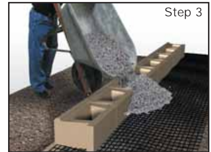
Backfill the blocks and behind the blocks.
