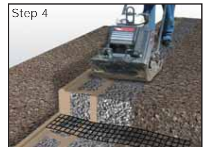
Backfill and compact, adjust for level as necessary.
