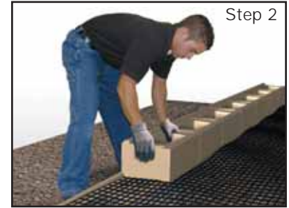
Place block on top of grid.
