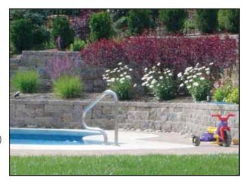
Plan ahead for walls that split into terraces. The area immediately behind the lower wall will require extra attention to ensure proper base preparation for the new wall above.
