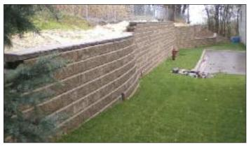
No-Fines concrete has been utilized in the construction industry for decades and the segmental retaining wall industry for more than 15 years. Like most concrete mixes, No-Fines concrete includes portland cement and coarse aggregate. However, sand (fine aggregate) is omitted from the No-Fines mix to allow voids
