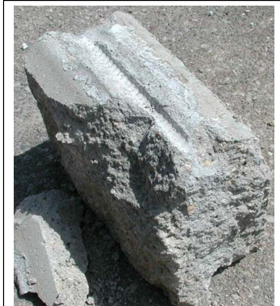
Figure 1: Sand Mix Grout in Panel
