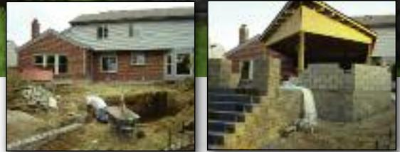
to install a retaining wall to create the raised patio the foundation of the project. Using Allan Block's Abbey Blend pattern, from the AB Europa Collection, along with 80 tons of backfill material the project had begun.
